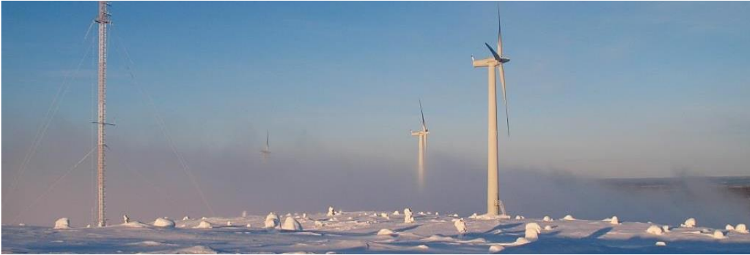
Figure 12: Olos fjell wind farm in Northern Finland (source: VTT)
