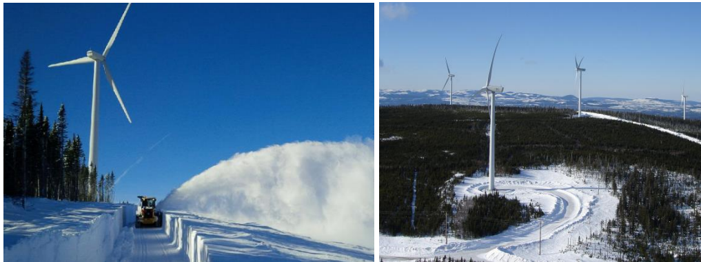
Figure 16: Snow removal allows for easy access to turbines with regular service vehicles but can be very expensive [318]
