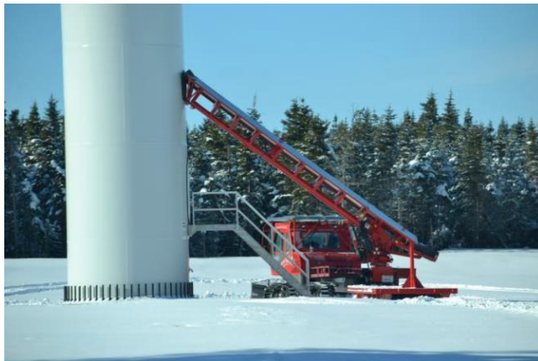
Figure 20: Mobile roof built by GDF Suez at Caribou wind parc to access wind turbines requiring maintenance when there is a risk of ice throw [321]
