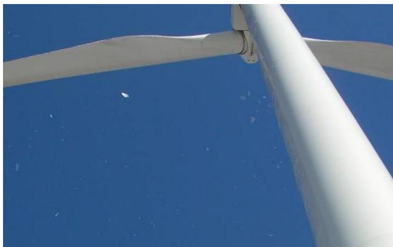
Figure 8-2-1: Ice falling or being thrown off a wind turbine poses a safety threat to turbine maintenance staff and, depending on turbine siting, the general public. Photo credit: Jeroen Van Dam, USA
