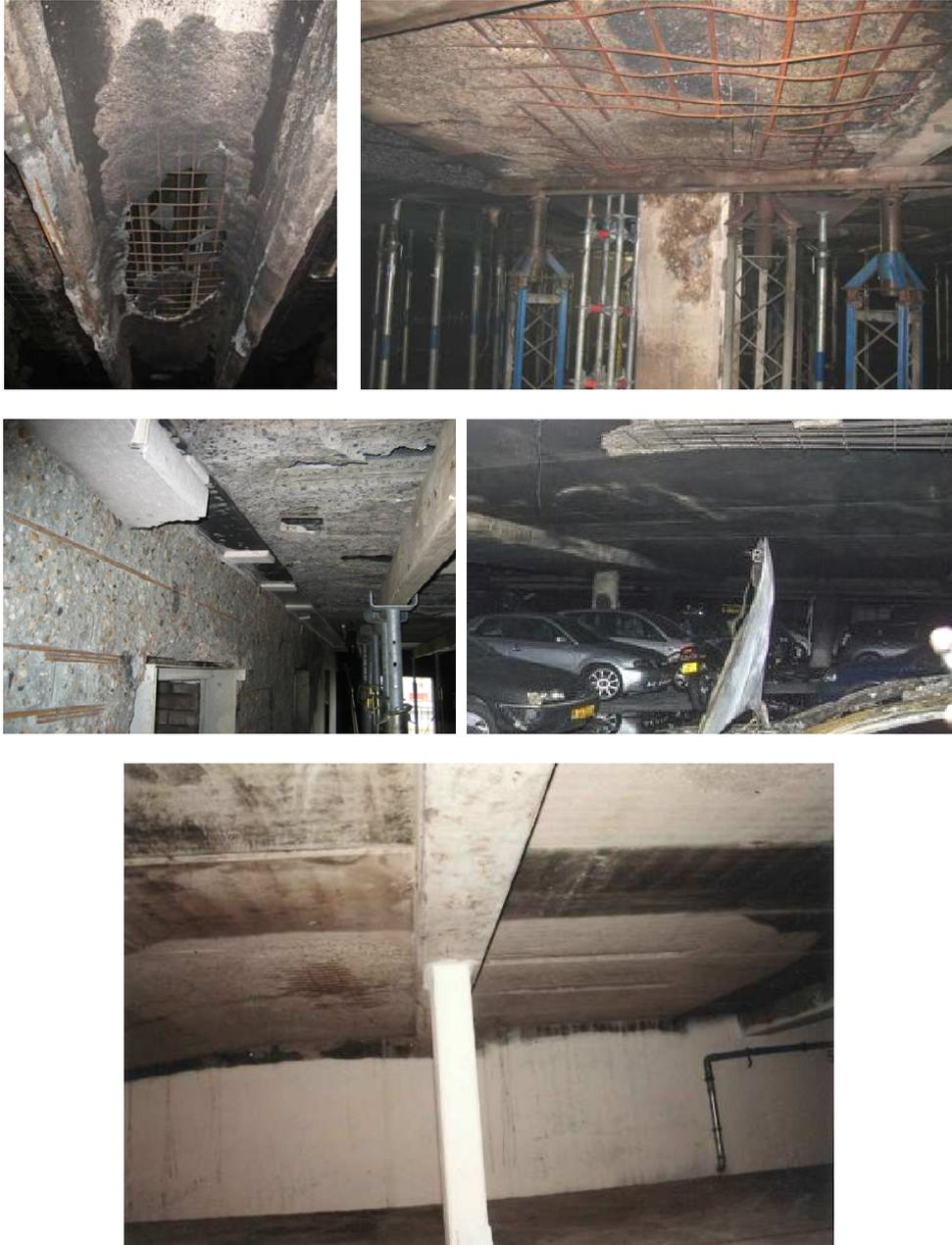
*Figure 7.29. Different concrete structures; same type of damage*
