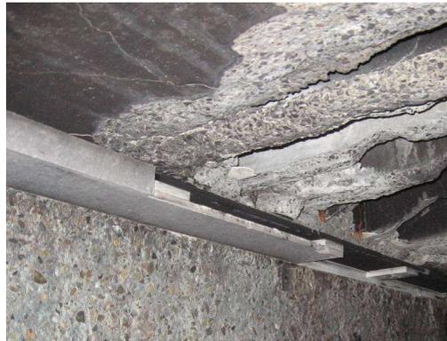
Figure 5.4-right. Support of the hollow core slab was intact
