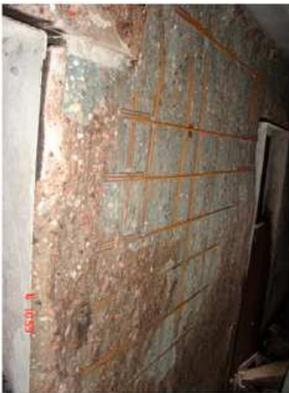
Figure 5.3-left. Extensive spalling on external facade surface
