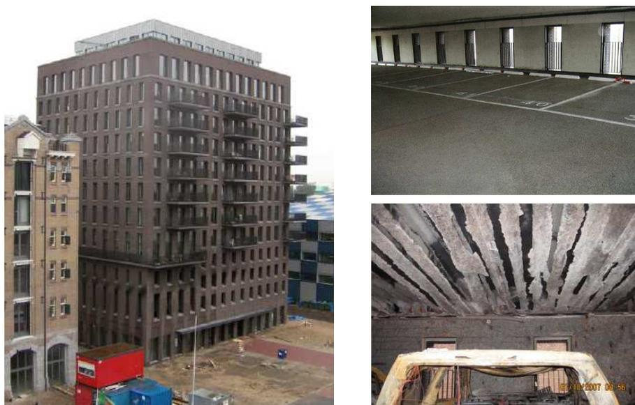
Figure 5.1. Building Harbour Edge in the Lloydstraat after fire (left). Level 3: intact floor above the fire where cars were removed the day after (right, top). Level 2: locally damaged ceiling above burned car on the level where the fire took place (right, bottom) [5.4]
