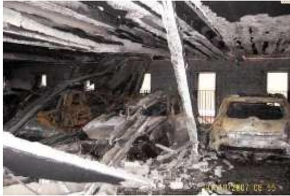
Figure 5.3-right. Hollow core floor ceiling with local damage, visible are cars 2, 1 and 3
