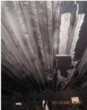
Figure 5.4-left. Underflanges of hollow cores felt down, and strands were exposed,
