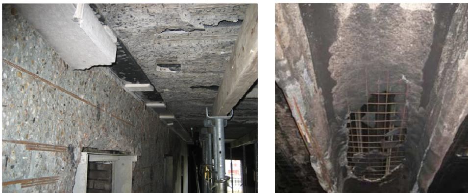
*Figure 7.1. Examples of buckling spalling combined with explosive spalling on walls and floors [7.1, 7.11]*
