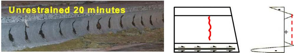
Figure 4.9. Vertical thermal cracks in hollow core slabs due to temperature gradient over cross section [4.14]
