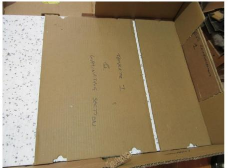
Adding the top laminating layer of cardboard to the polystyrene sheet. Note the initial half-section at the end of the box, to ensure that joints are staggered in all layers of the structure as you assemble the 3 boxes.
