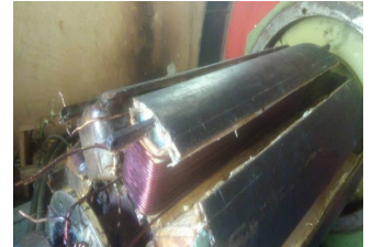
re-wound pole on generator rotor
