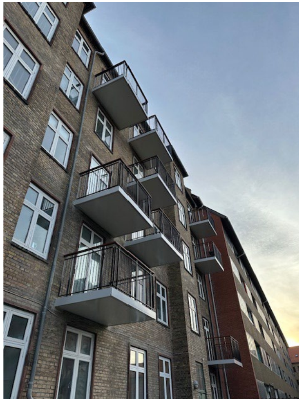
Figur 12 - altaner mod baggård
