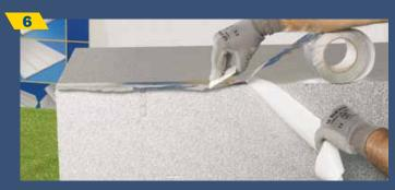
Using the nylon marking pencil, the dimensions of each duct can be easily traced
