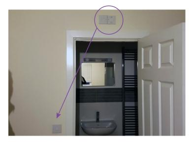
the client has requested that the isolator switch that is above the door be moved to the same position as the light switch.
