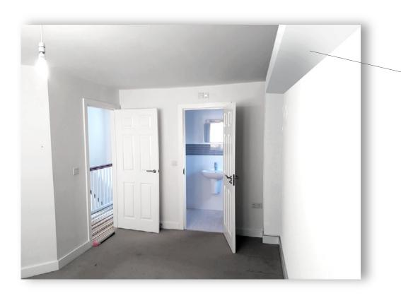
New lighting bulkhead - same width and depth of soil stack 215 x 215mm to span the length of the room 4240mm (from soil stack)
