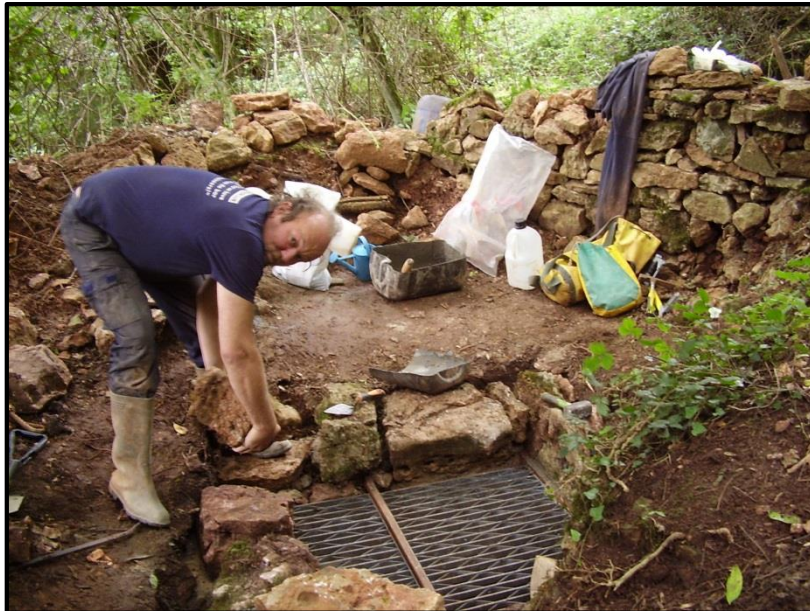
Alex working on the new entrance.
