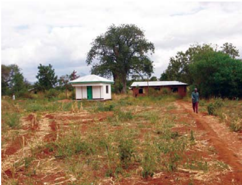
The health facility constructed in Tanzania, Moshi District – still awaiting staff and funds for recurrent costs. The missing linkages between community/ political planning (whether through Local Government (LG) structures or CDF) and technical health district planning are found in all 3 countries. While probably most significant in Kenya it is still serious in Uganda and Tanzania.
