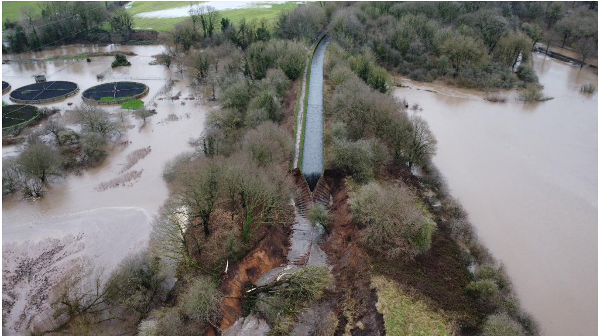
Bridgewater Canal breach January 2025 (credit Taylors Aboard)
