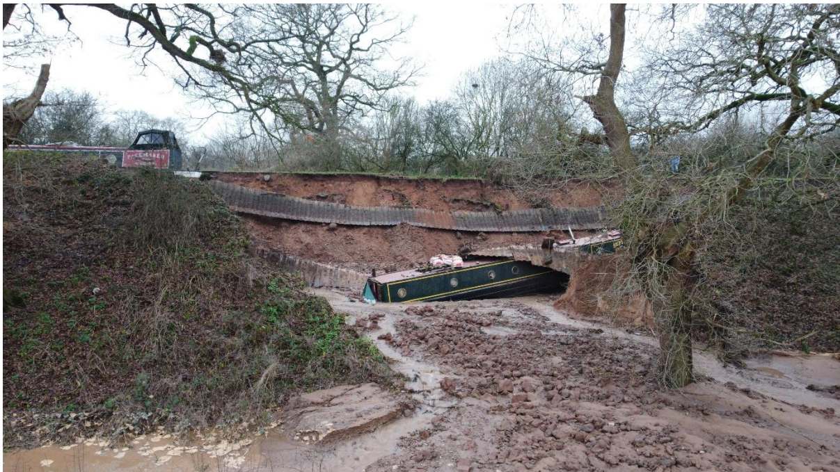
Llangollen Canal breach December 2025 (credit Taylors Aboard)
