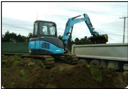
Traditional digger with track
