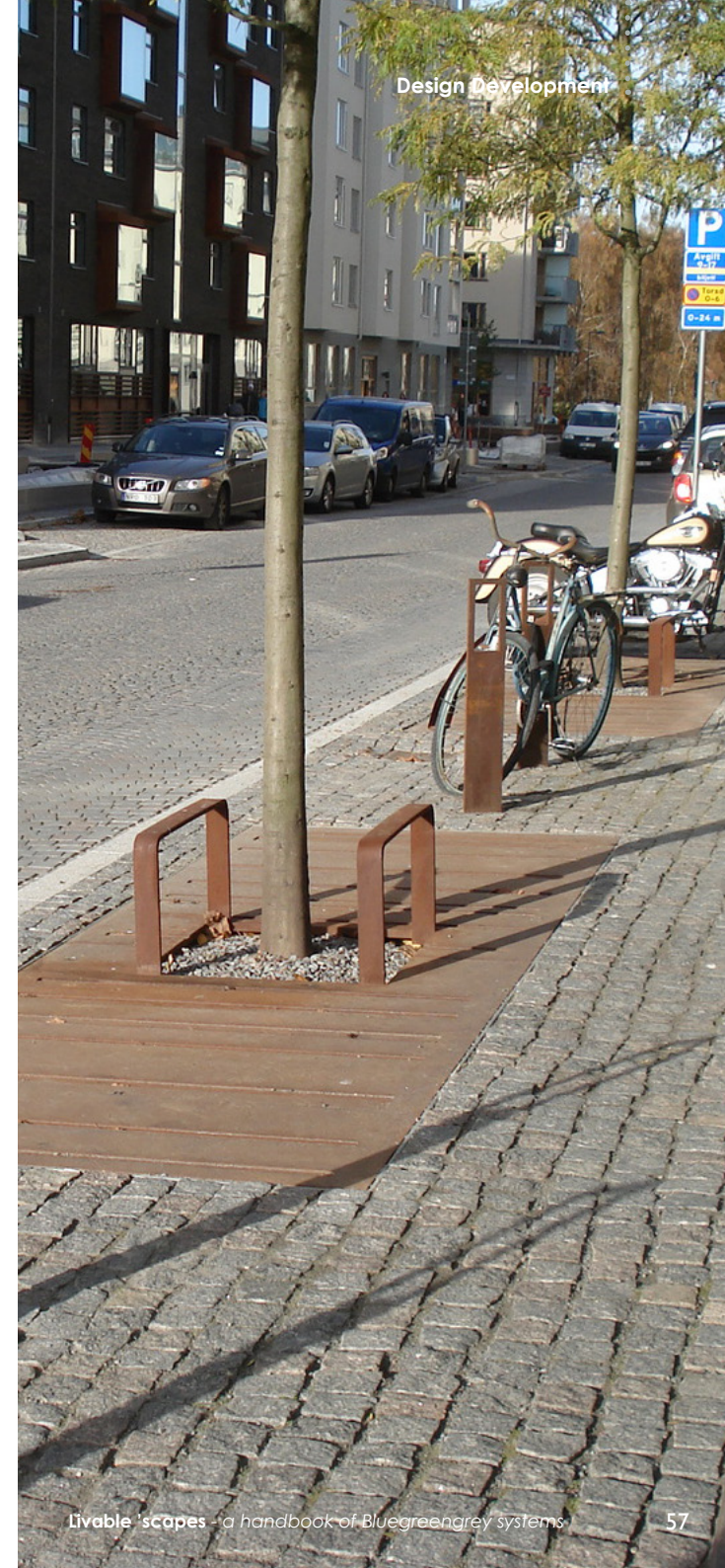
▲ Figure 33. Covered bioretention area on open subbase layer in generally lower-demand conditions.
