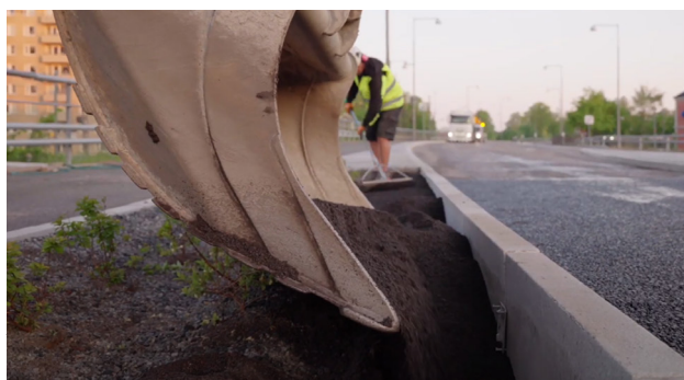
▲ A plantbed that has direct connection to curbstone after application of Locstone.
