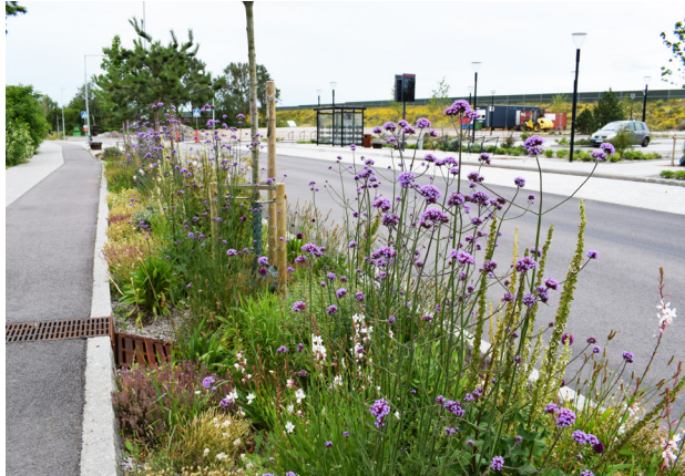
▲ Bioretention area and hard surfaces on a strip of open subbase layer. Campus area, Vellinge.
