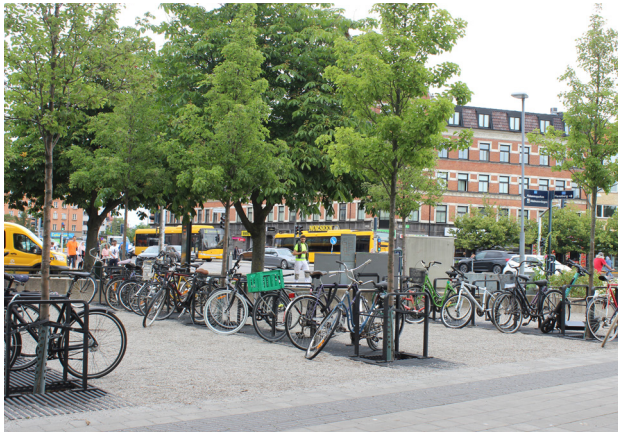
▲ Bicycle parking with permeable pavements on open subbase layer which acts as a water reservoir for stormwater and green space. Södervärn, Malmö.
