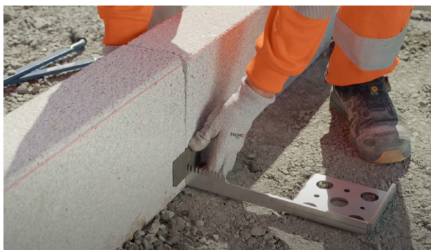
▲ An example of application of Locstone that holds together blocks of curbstone without usage of concrete.
