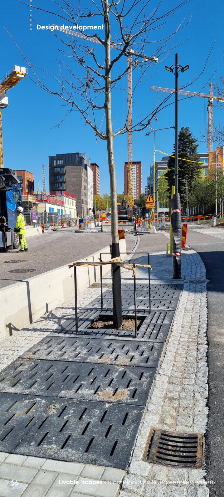
◀ Covered bioretention area on open subbase layer. Nacka. Foto: Agata Wehlin.
