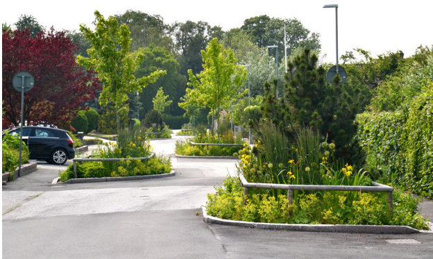
▲ Separate bioretention area on open subbase layer. Rundelsgatan, Vellinge.
