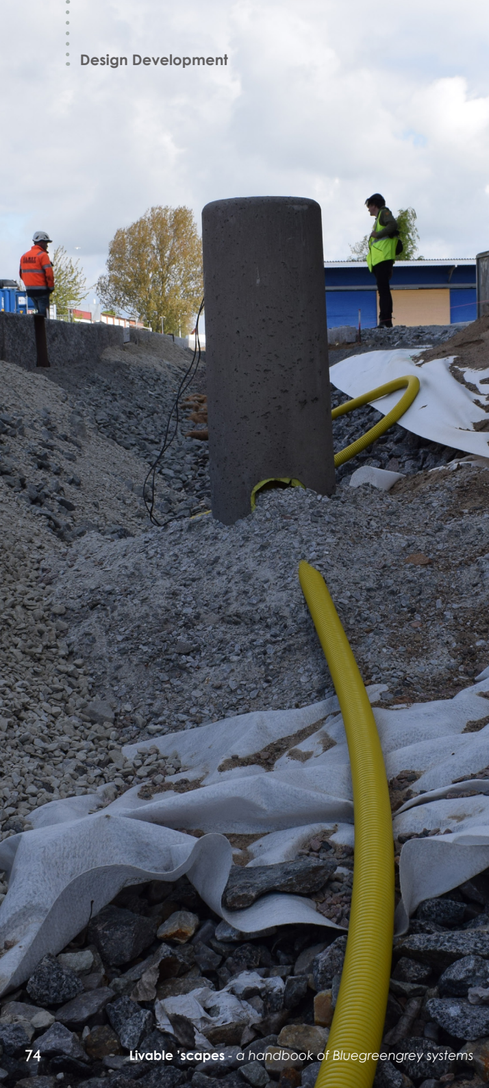
◀ Construction of BGG-system Norra infarten, Vellinge
