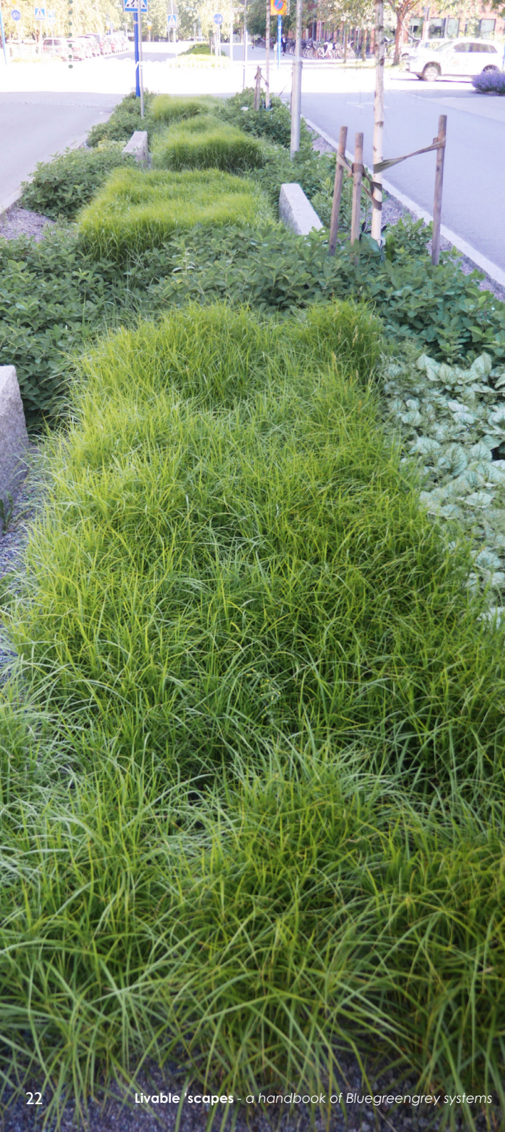
◀ Bioretention area on the street Strandbogatan, Uppsala. Photo: Rasmus Elleby.
