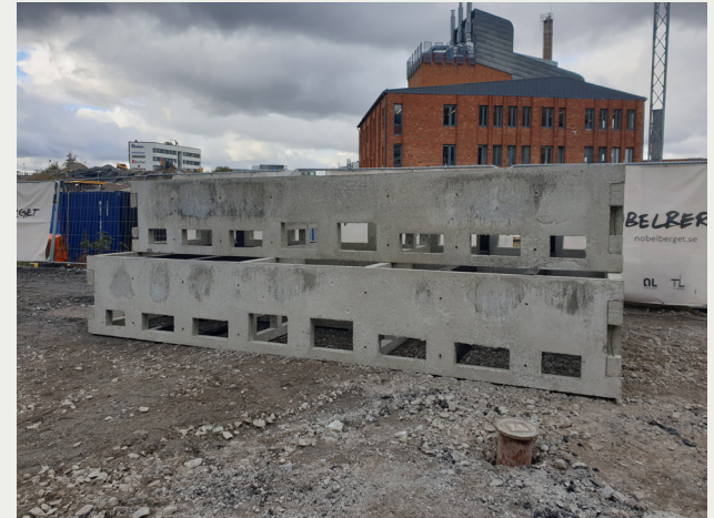
Concrete frame for covered bioretention area. Foto: Agata Wehlin
