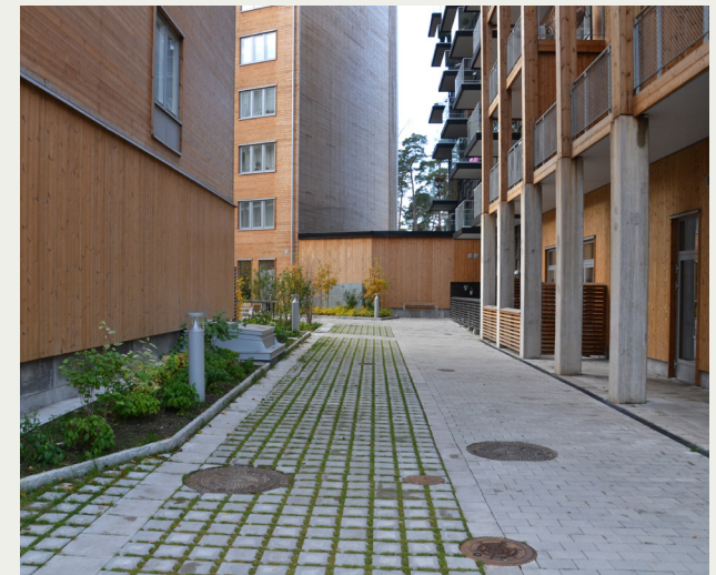
Permeable hard surface on open subbase layer with joints of grass on residential land. Rosendal, Uppsala.
