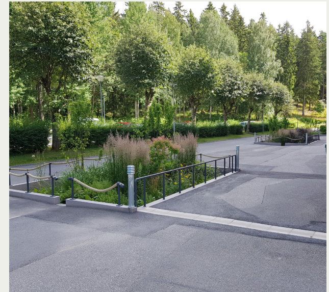
Rain bed on neighborhood land that takes care of stormwater from surrounding asphalt surfaces and roofs. Södertälje. Photo: Fredrik Ohls.
