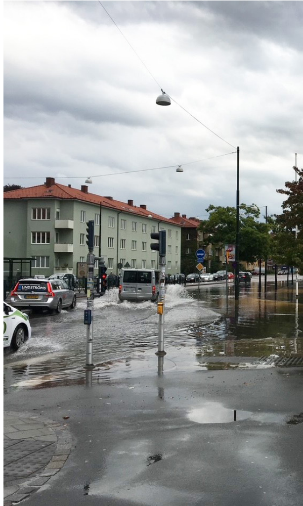
▲ Flooding of hard surfaces with conventional construction and stormwater management. Folkets park, Malmö.
