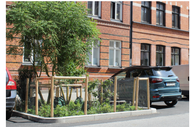
▲ Parking spaces and bioretention area on a strip of open subbase layer. Ängelholmsgatan, Malmö.
