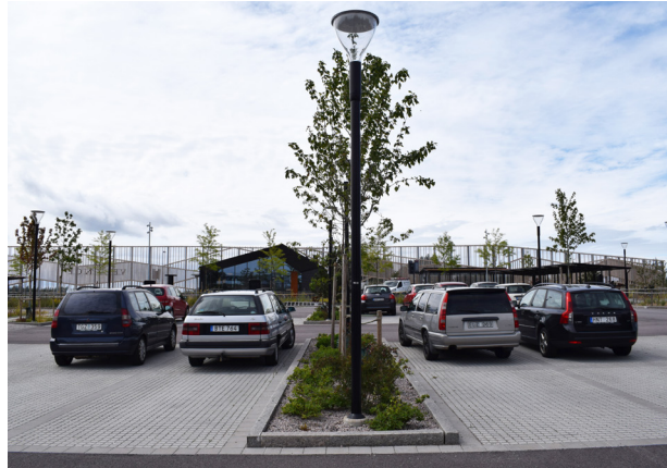
▲ Permeable pavement and vegetation area installed on open subbase layer. Campus area, Vellinge.
