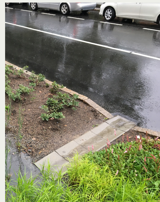
Inlet with lowered curb edge. Strandbogatan, Uppsala. Foto: Rasmus Elleby
