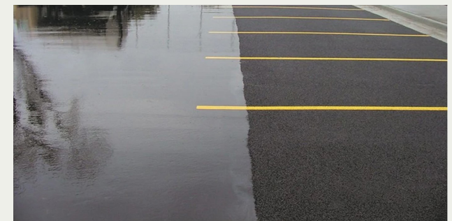
Impermeable and permeable hard surface made of asphalt.
