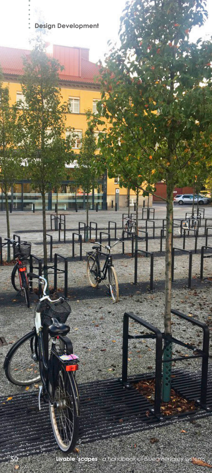
◀ Bicycle parking with open subbase layer. The entire superstructure under this area serves as a planting bed and stormwater reservoir. Södervärn, Malmö.
