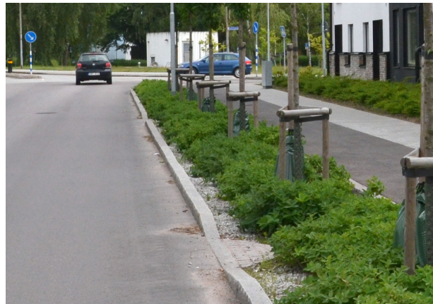
▲ Narrow and shallow bioretention areas as well as bicycle lane and pedestrian walkway on open subbase layer. Perstorpsgratan, Vellinge.
