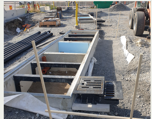
Covered bioretention area under construction, Nacka. Foto: Agata Wehlin.
