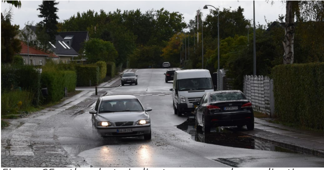
Figure 65 – the photo indicates one weak canalisation node on Rybjerg Alle during a very short cloudburst.
