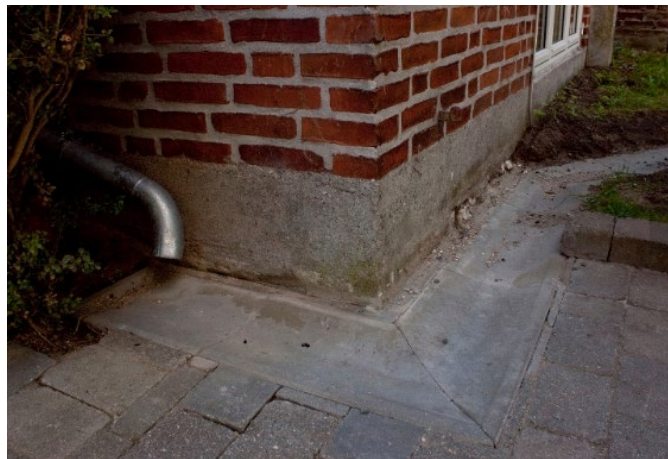
Figure 33 - a detail view on the gully and disconnected downpipe
