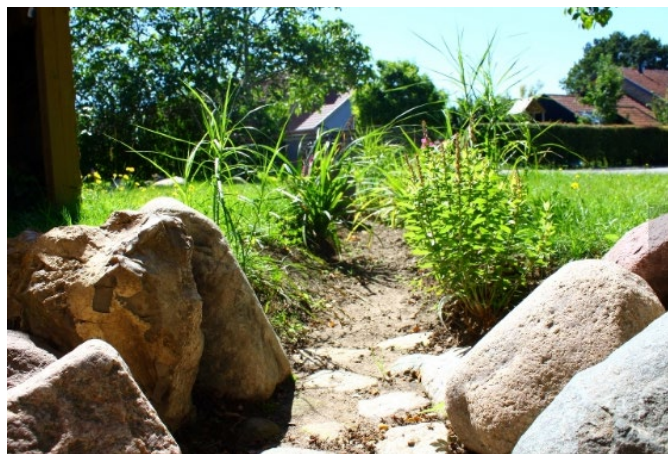
Figure 34 - the bioswale that transports rainwater from the gully into the rain garden
