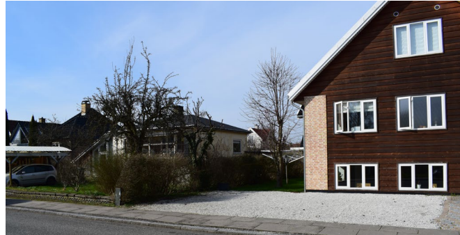
Figure 70 – use of crushed stone can partly preserve the function of soil to infiltrate rain water while the owners can still use it for parking their cars
