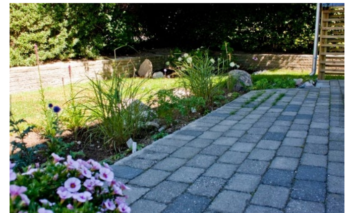
Figure 39 - the rain garden collects rain water from the storm water planter. During heavy rain the excess rain water from the rain garden can overflow into a nearby dry basin.
