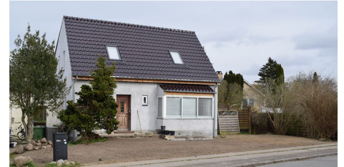
Figure 74 – opposite approach from the previous photo. The owner - who personally provided information about his intentions during on-site research – is creating in front of the house a smooth, steep slope up towards the house to protect it against floods that might reach the house from the street. In his back garden, he uses soak-aways to retain and infiltrate rain water from another side of the roof.
