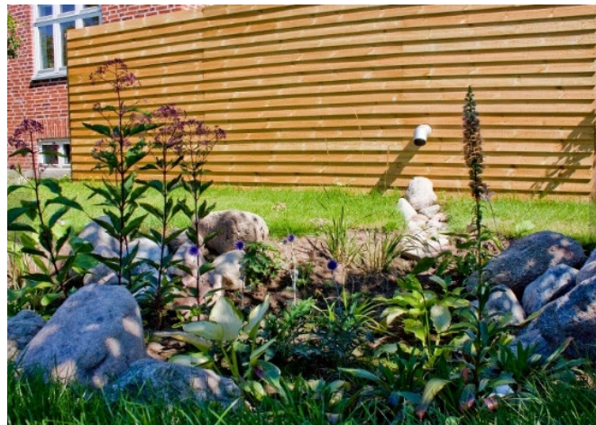
Figure 35 - a photo of the rain garden that collects rain water together with a view on a second downpipe with the gully in a background
