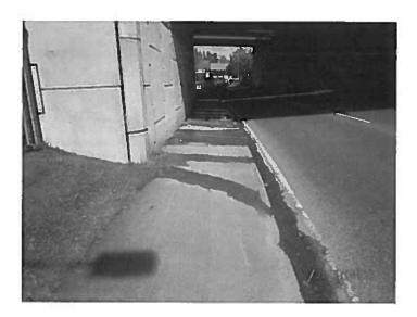
2.4 CMS have been instructed to carryout weekly monitoring of the surface of the road and the face of the retaining wall. To date no significant further movement has been noted.
