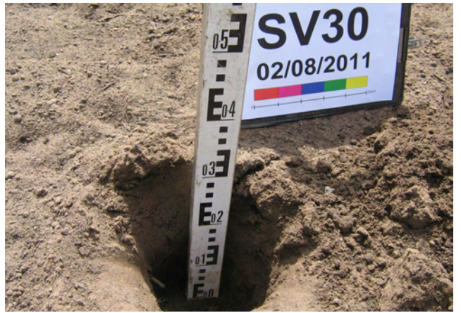
6. SV30 verification of topsoil depth with school landscaping – 300mm deep.
