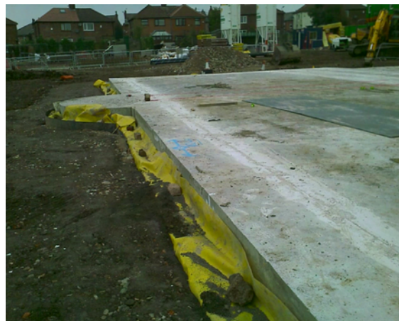
Gas Membrane (yellow sheet) with joint sealed Insulation above membrane (left of photo) Slip Sheet above insulation (right of photo) Preparation for concrete pour showing reinforcement (far right of photo)
