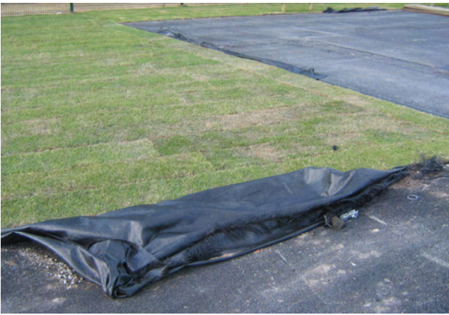
9. Landscaping in the west of site, membrane visible
