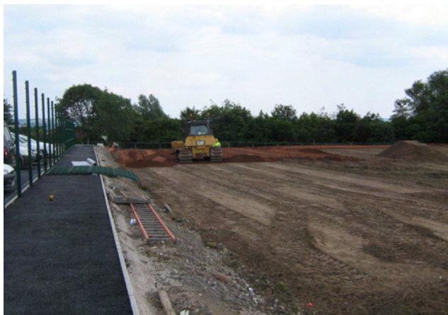
3. Import of topsoil and sand for pitch area July 2011
