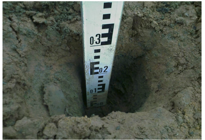
4. SV10 verification of topsoil depth within football pitch – 300mm deep (18/07/11).
