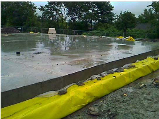
Gas Membrane (yellow sheet) with joint sealed Insulation above membrane (left of photo) Slip Sheet above insulation (right of photo) Preparation for concrete pour showing reinforcement (far right of photo)
