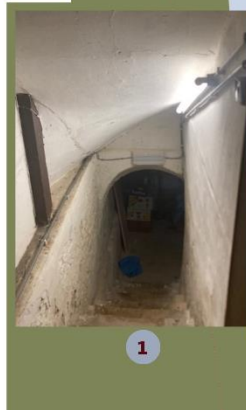
[basement stairs] 02-ground floor
