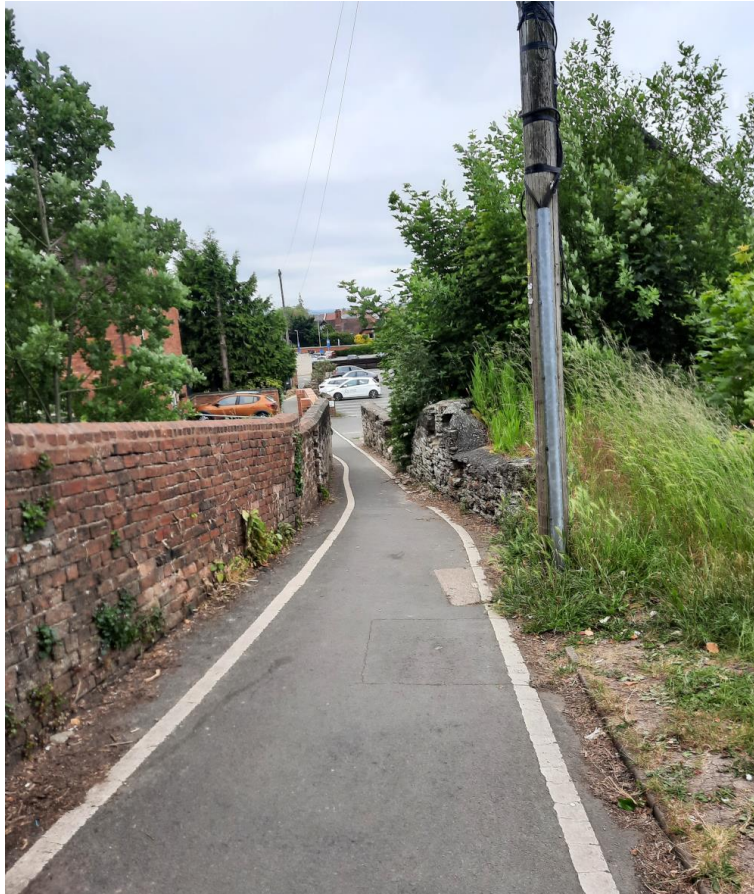
Figure 19. Narrows on Portcullis Lane (early morning image)
