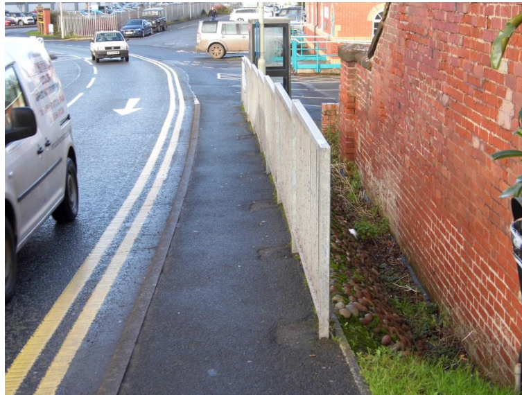
Figure 21. Narrow pavement south of station
