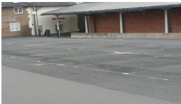
Eroded lines and missing signage in Upper Galdeford car park
