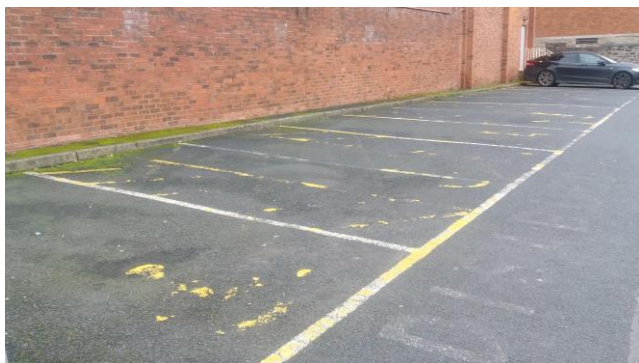
Eroded lines and missing signage in Upper Galdeford car park
